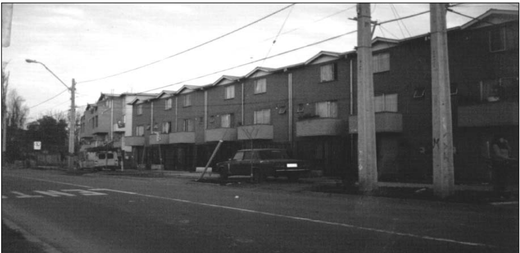
Figure 4. Social housing in Villa Nueva Resbalón, in the municipality of Cerro Navia, Santiago (2005)
